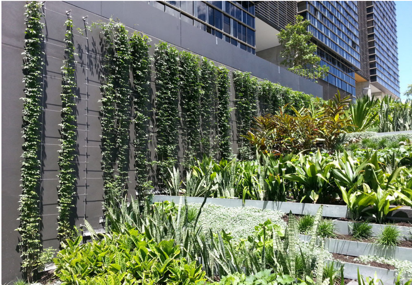
Vertical Tensile Wires and cross beams create green columns up vertical surfaces Image supplied by Tensile Design & Construct.
