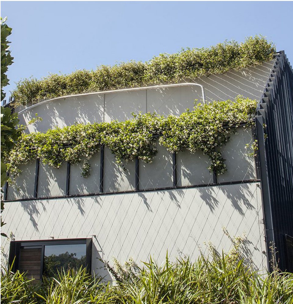
Image supplied by Tensile Design & Construct. Project: Anderson Rd, Melbourne Wall: East Facing
